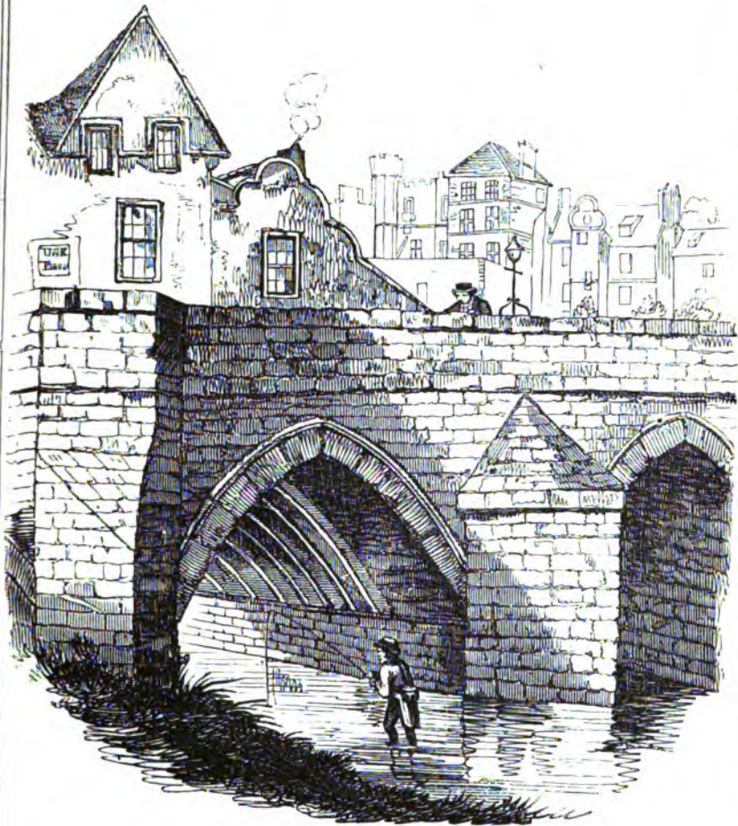
ELVET BRIDGE, DURHAM.
